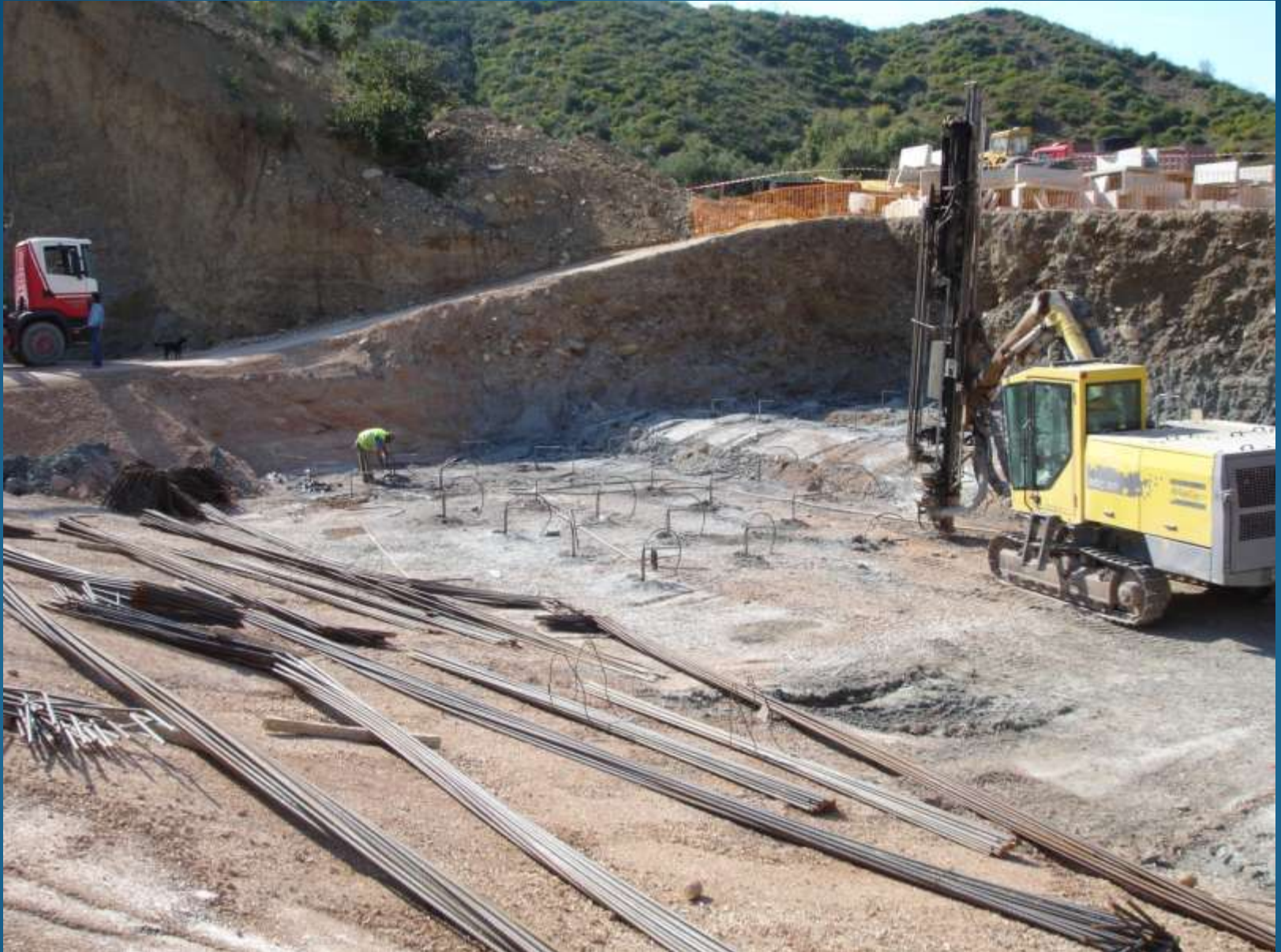
Anchors on the bottom of the spillway
