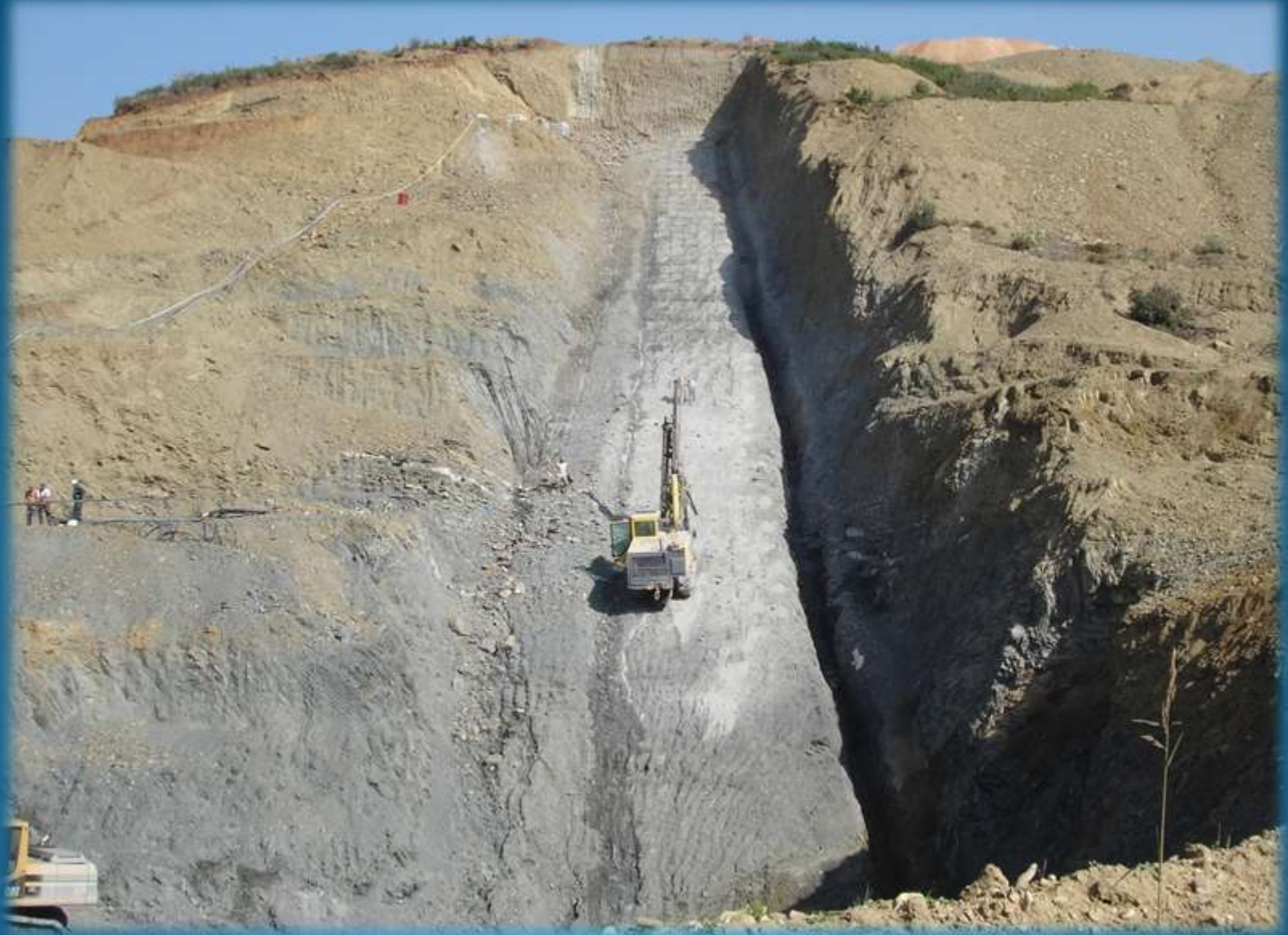
Drilling for the plinth anchors
