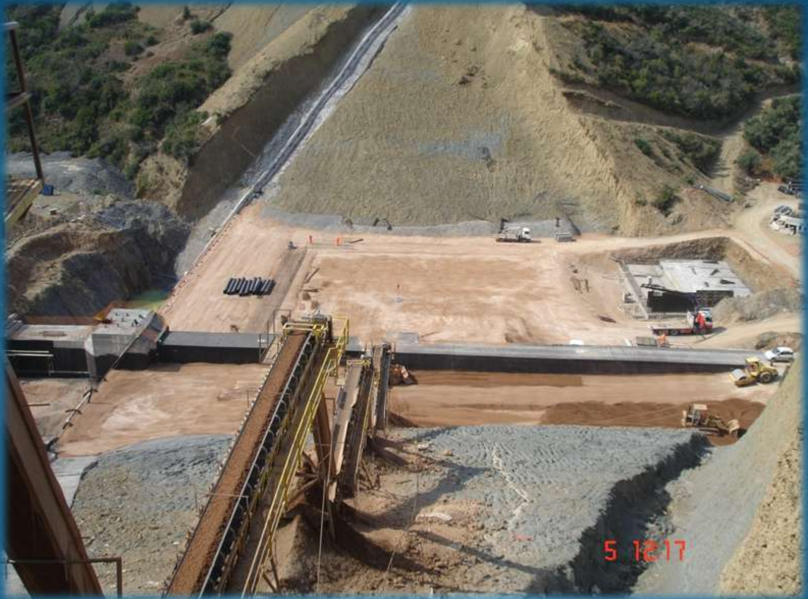
Building the drainage culvert
