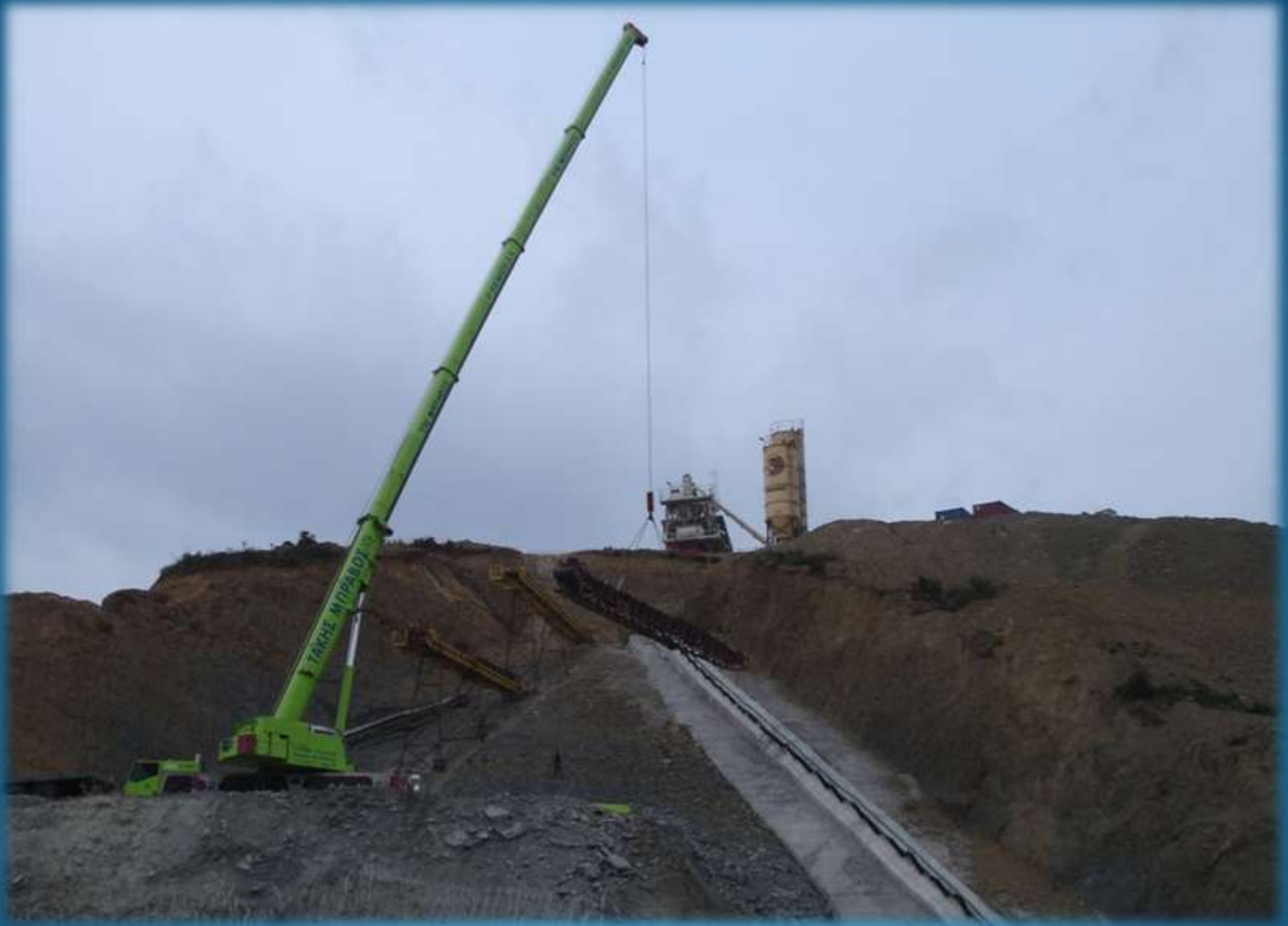
Installation of belt conveyors
