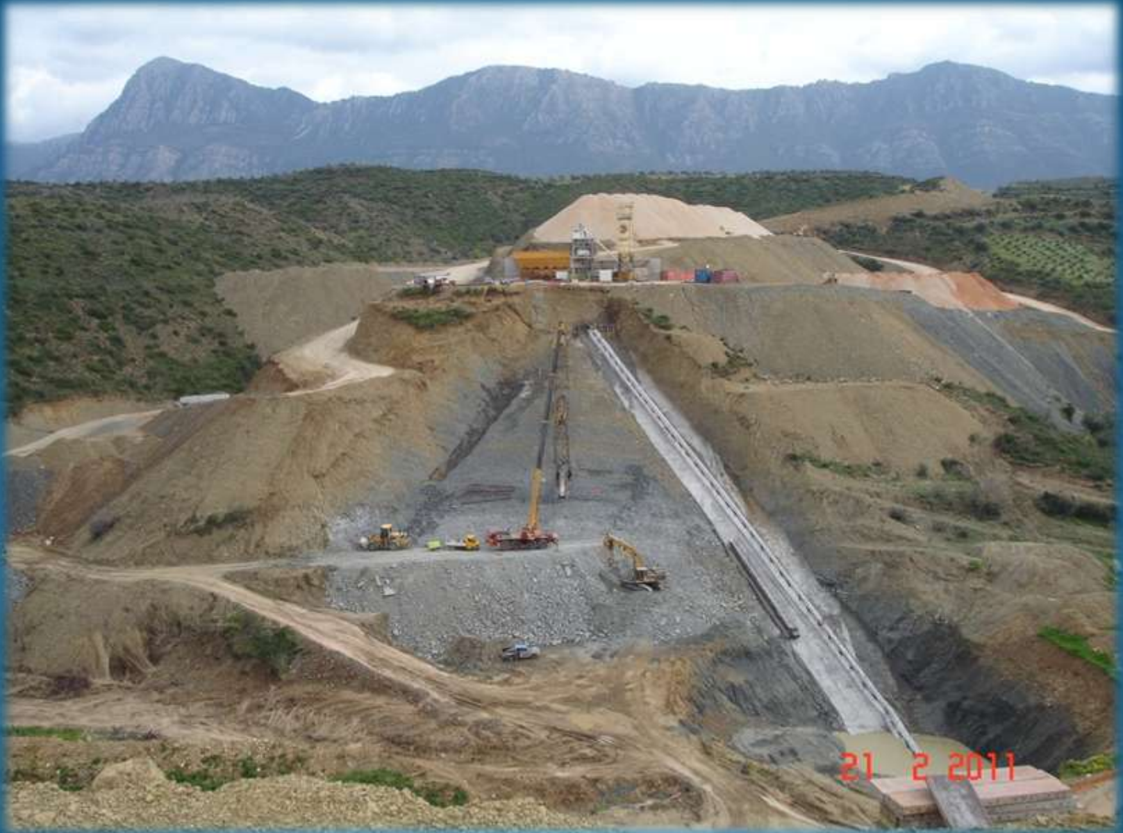
Installation of belt conveyors
