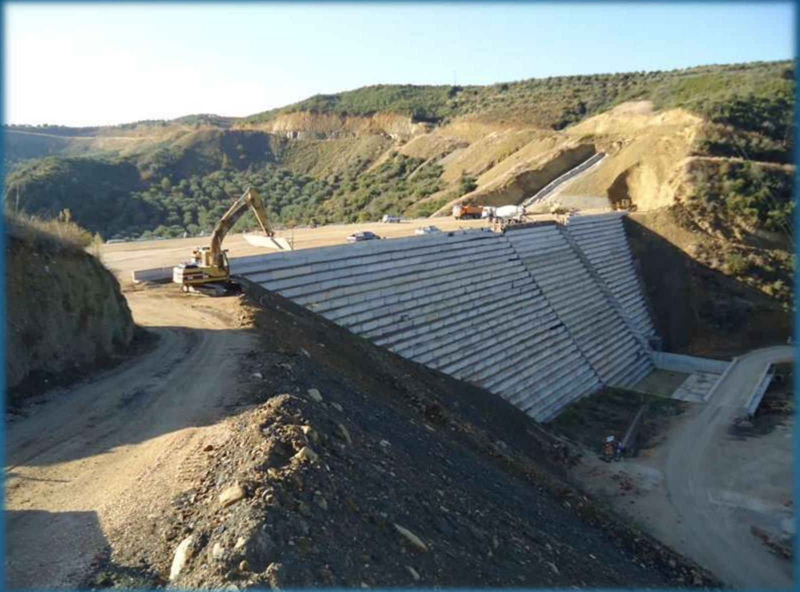
Downstream steps and the spillway
