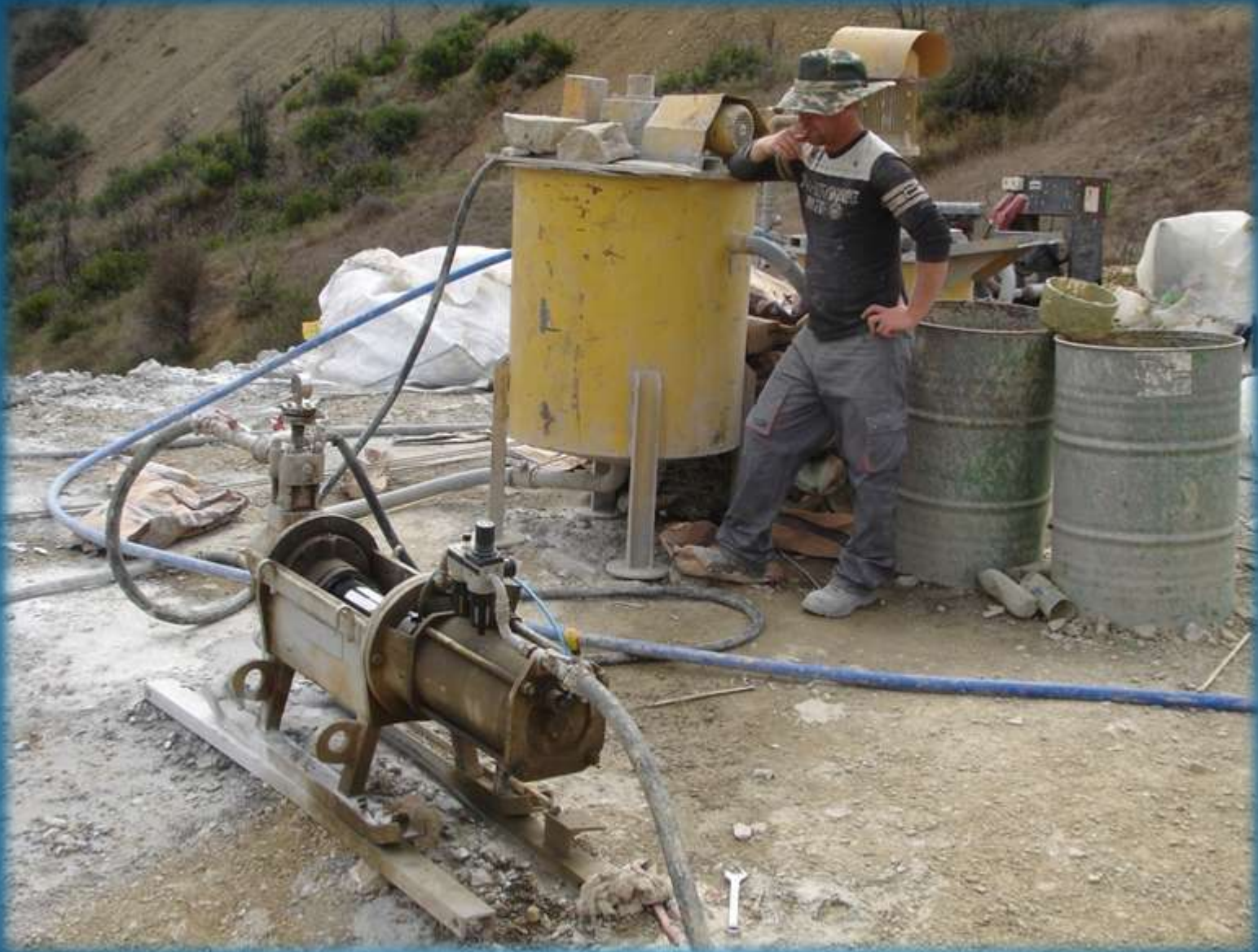
Cement grouting
