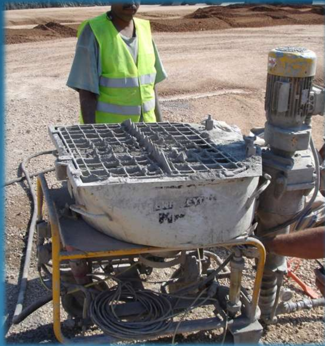
Grouting the anchors
