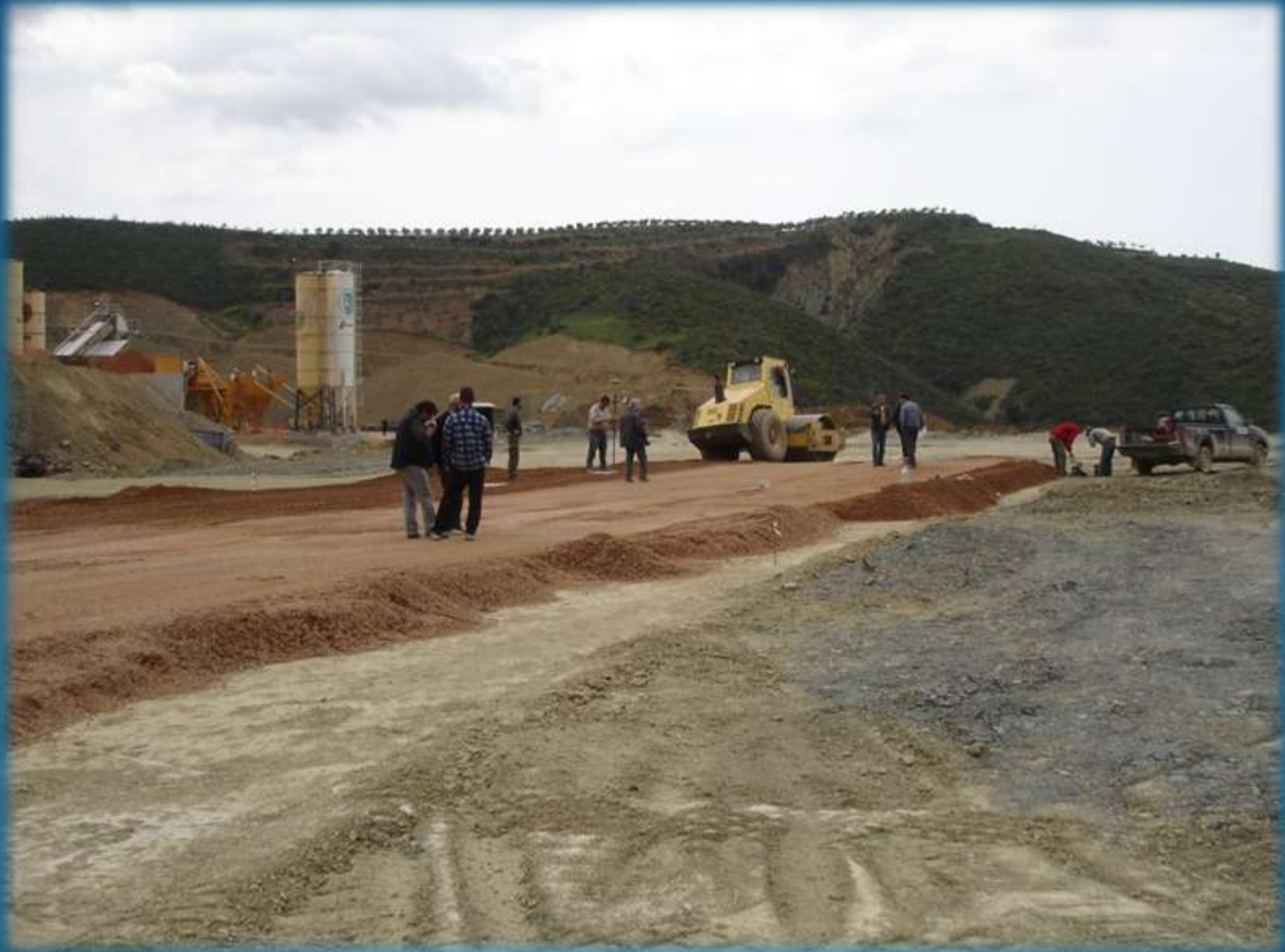
Trial test section (by lean RCC)
