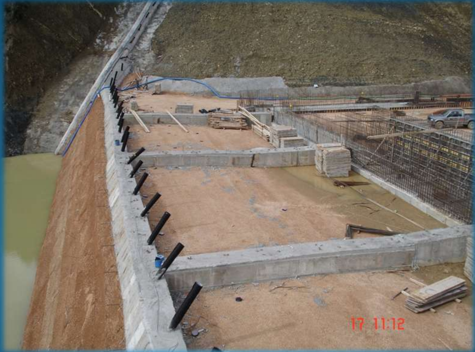
The main upper drainage pipe
