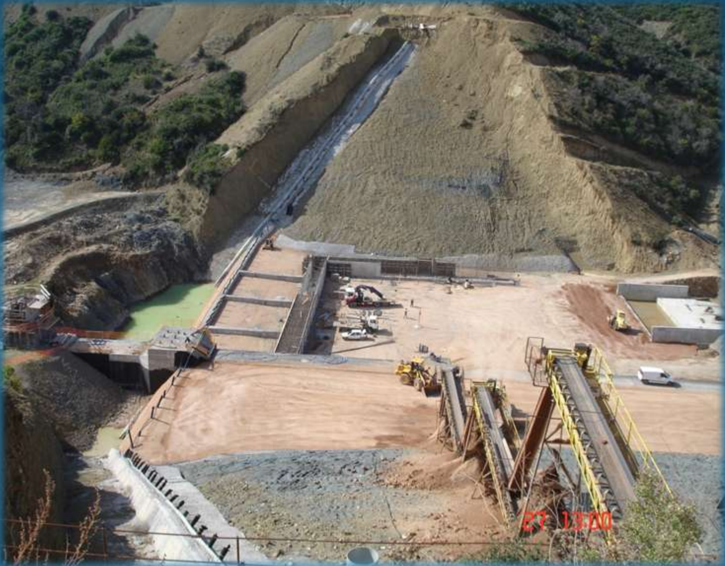
Building the drainage culvert
