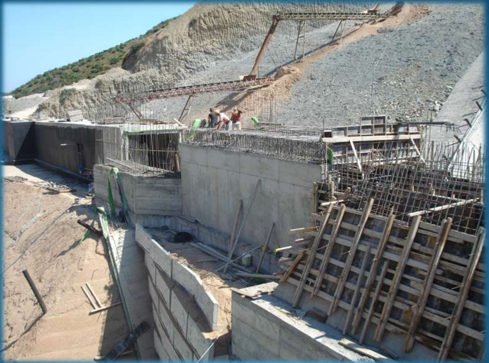
Box culvert for the final diversion of the river
